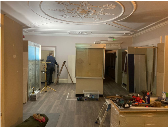
The more measured “Nigel” approach.
